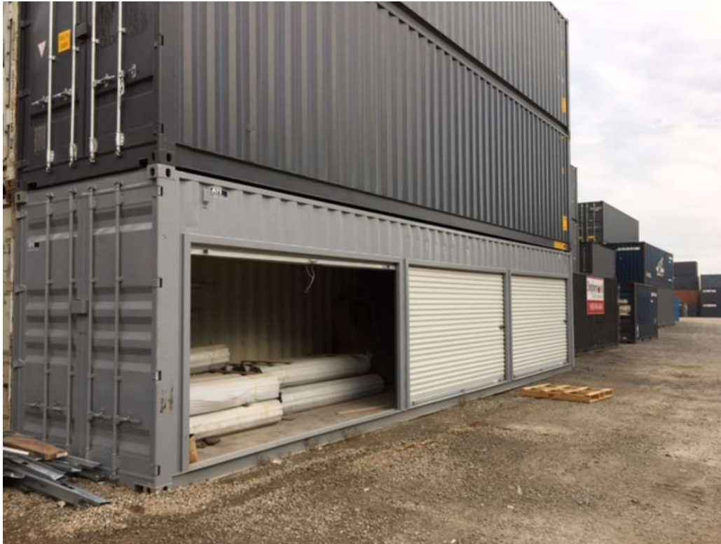
Figure 4 – Sea Can Container Barrier
