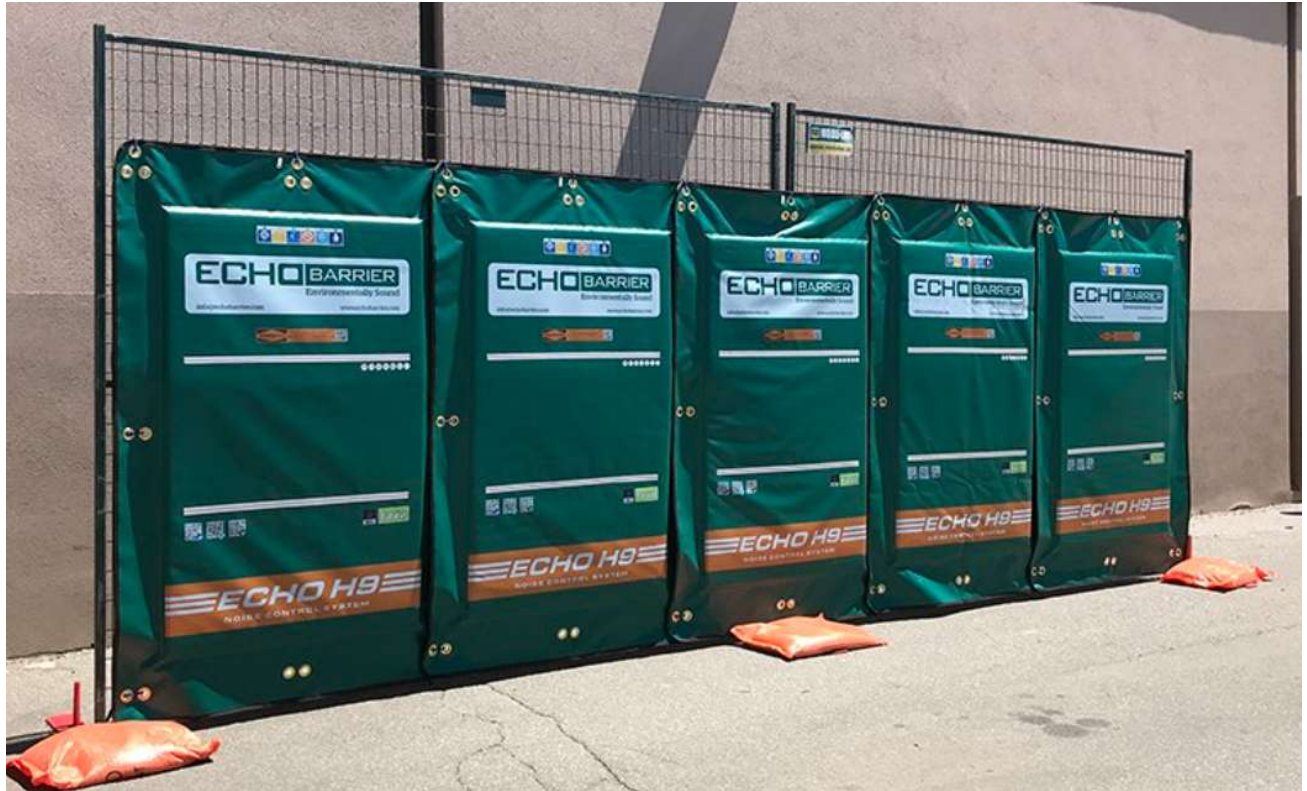
Figure 6 – Echo H9 Loaded Vinyl Sheets on Mesh Fence
